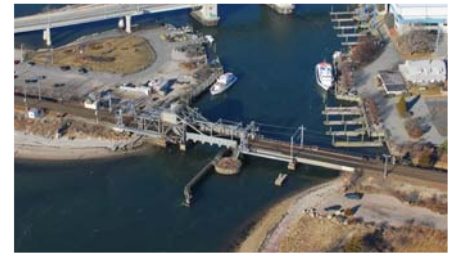
The Span at Niantic River before renovation.
