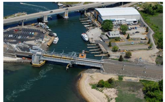
The completed bridge at Niantic River.
