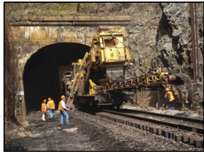
Lowering track at Eggleston Tunnel in Virginia
