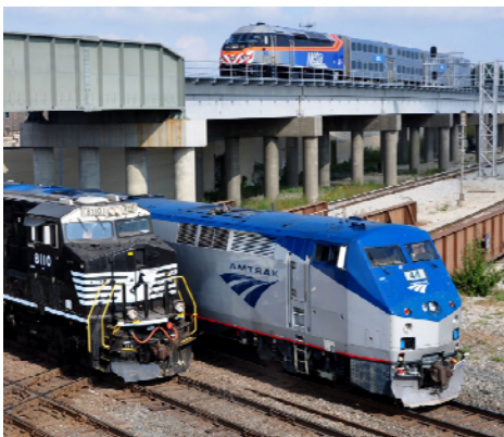
New Metra Rail Bridge over Norfolk Southern tracks
