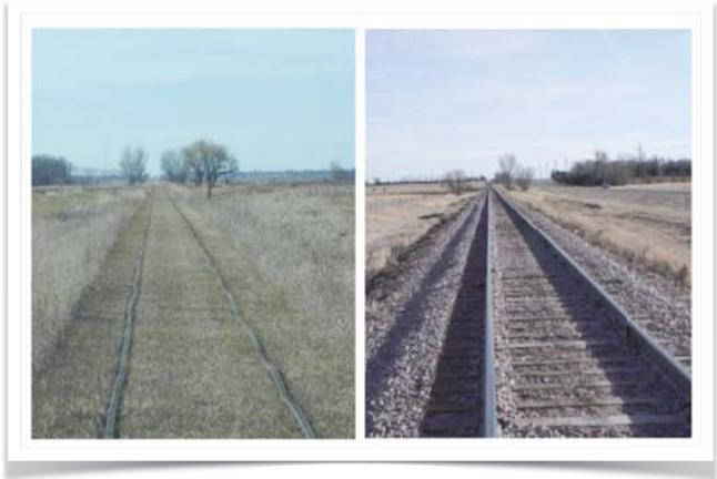
Track conditions at milepost 4 in 2010 and 2012, before and after the completion of the USDOT TIGER II Project.
